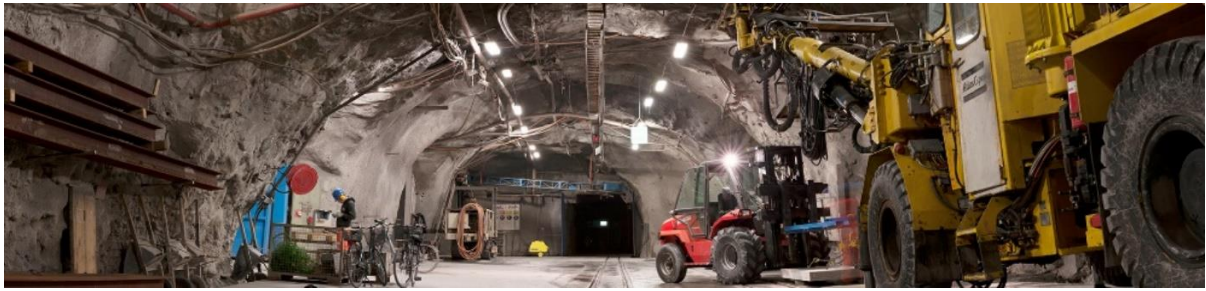
Picture 2: Highway Profile of the Hagerbach Test Gallery
